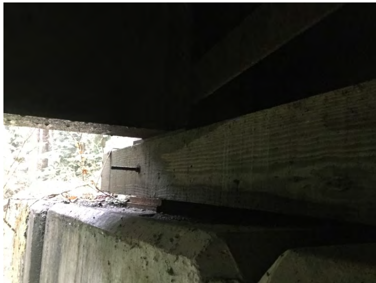
Downstream right bank timber sill shimmed
