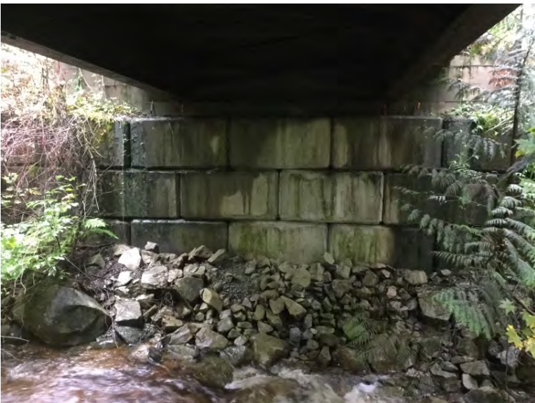
Left Bank Abutment when facing downstream
