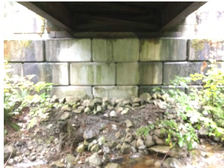
Right Bank Abutment when facing downstream
